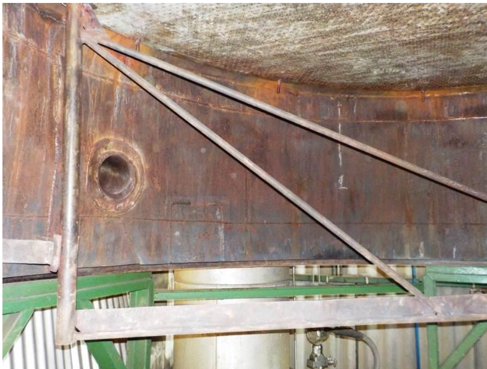
Photo 2: Internal part of the R-1101 Reactor Cover.
