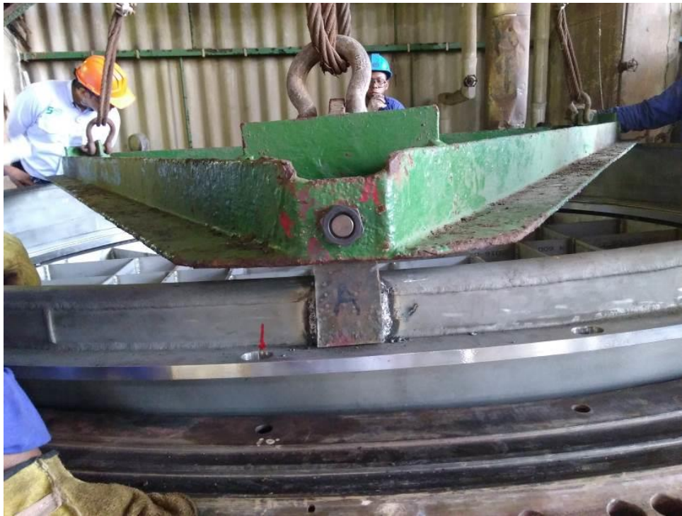
Photo 1: Attachment point - Flanged connection of the basket to Reactor R1101
